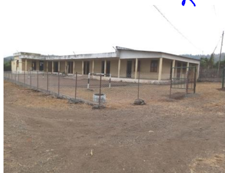
Primary School, Marapadol with fencing, gate with lock and khidki
